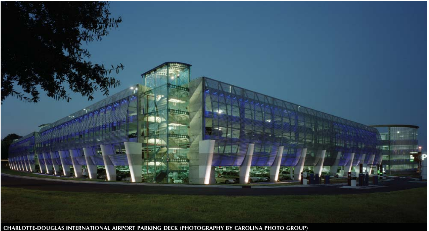
CHARLOTTE-DOUGLAS INTERNATIONAL AIRPORT PARKING DECK (PHOTOGRAPHY BY CAROLINA PHOTO GROUP)
