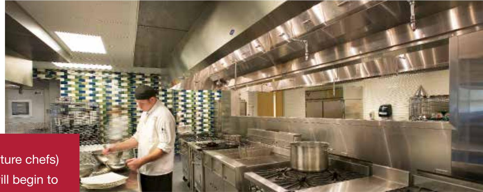
facilities will be ready for anything that technology is able to cook up next. Bing and Sousa utilized utility distribution systems (UDS) throughout the kitchens that allow quick disconnects and replacements for kitchen equipment without expensive, time-consuming rewiring and repiping of electrical and gas connections. Other common-sense strategies such as high, clear structural spans accommodate adaptability and ease of relocating equipment as necessary.
